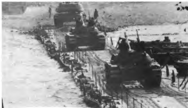
Figure 6-50. PMP heavy folding bridge. This new-type "ribbon bridge" provides a rapid-assembly heavy (class 60) bridge. The sections are carried folded on the backs of trucks. The trucks back up to the water's edge and dump their spans which open automatically as they hit the water. The bridge is assembled in the water along the shoreline and positioned by power boats.
